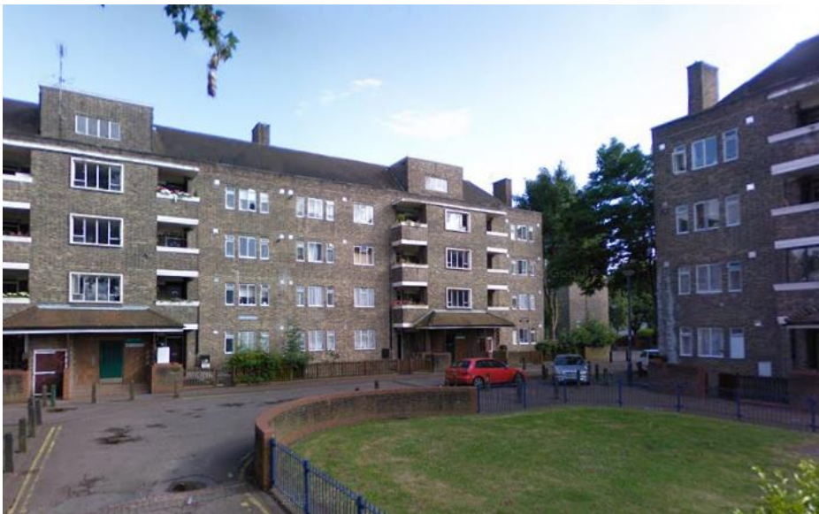
Image 3: View of the inside of Brecknock Estate viewed from the central walkway
