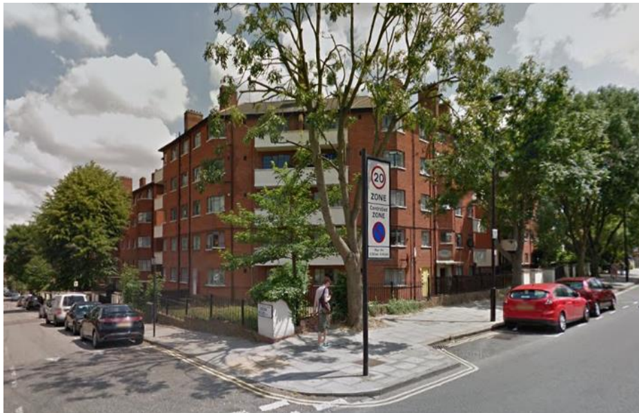
Image 1: View looking south east from the corner of Brecknock Road and Anson Road (Morris House)
